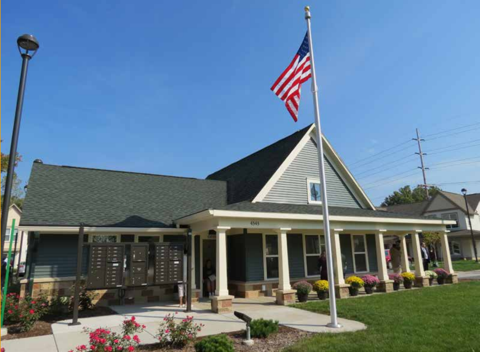
Photo: Courtesy of Genesis Non Profit Housing Corporation Genesis Woods apartments received LEED Gold Green Building certification from the U.S. Green Building Council.
